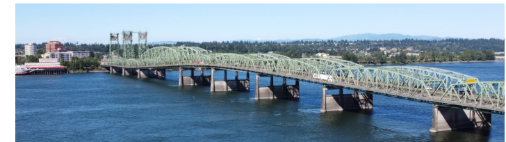
104-year old I-5 Bridge
