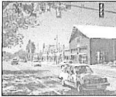
Distinct building presence on the street
