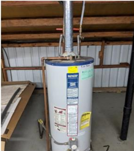
Figure 4.14. Building C Domestic Water Heater
