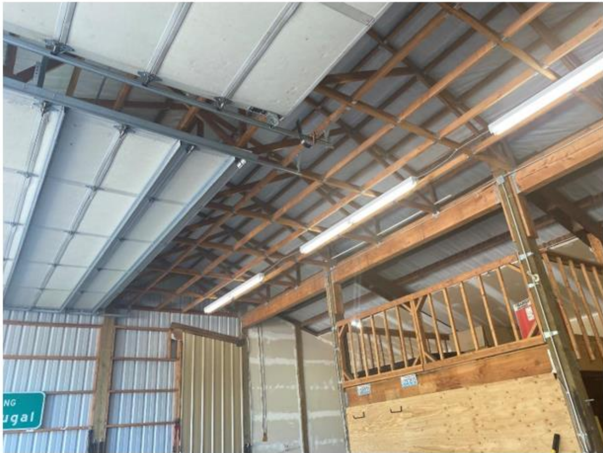
Figure 2.19. Building E Structure
