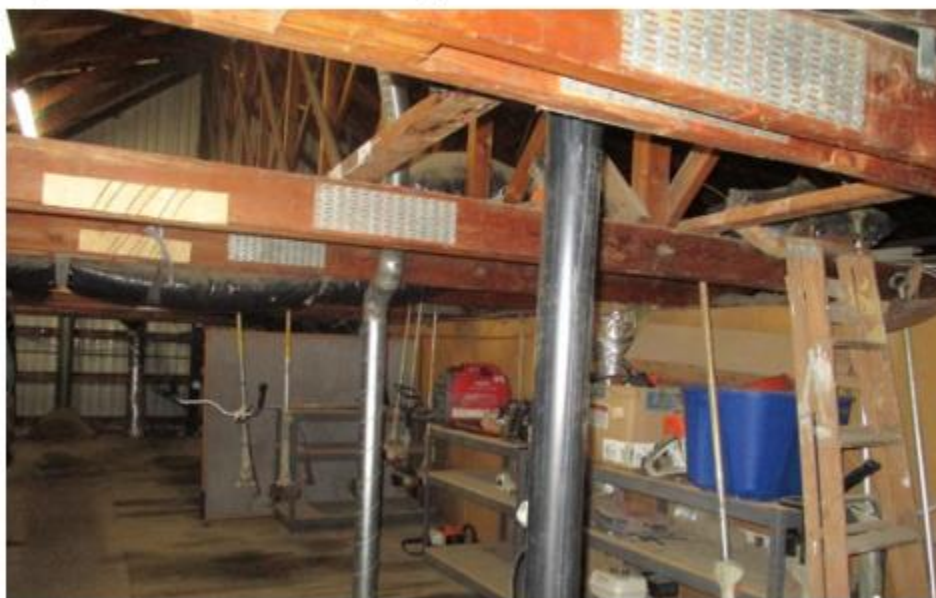
Figure 2.6. Area Used for Storage
