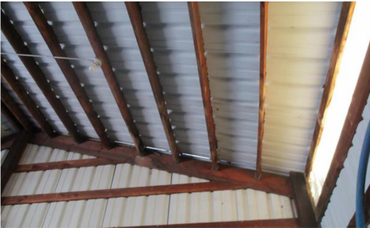
Figure 2.9. Gap at Edge of Roof
