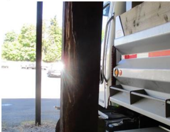
Figure 2.11. Column Damage
