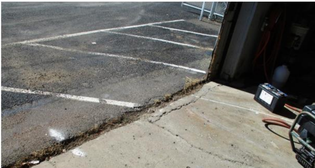
Figure 2.2. Example of Transition Between Asphalt and Concrete
