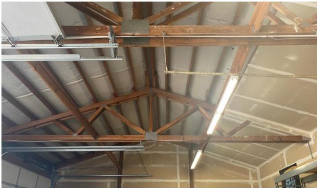
Figure 2.16. East Timber Trusses
