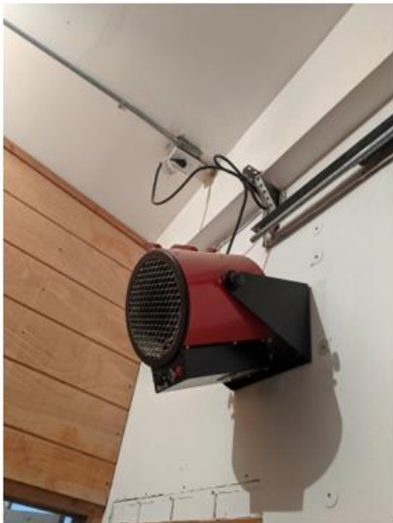
Figure 4.20. Building F Electric Unit Heater in Shop and Storage Area
