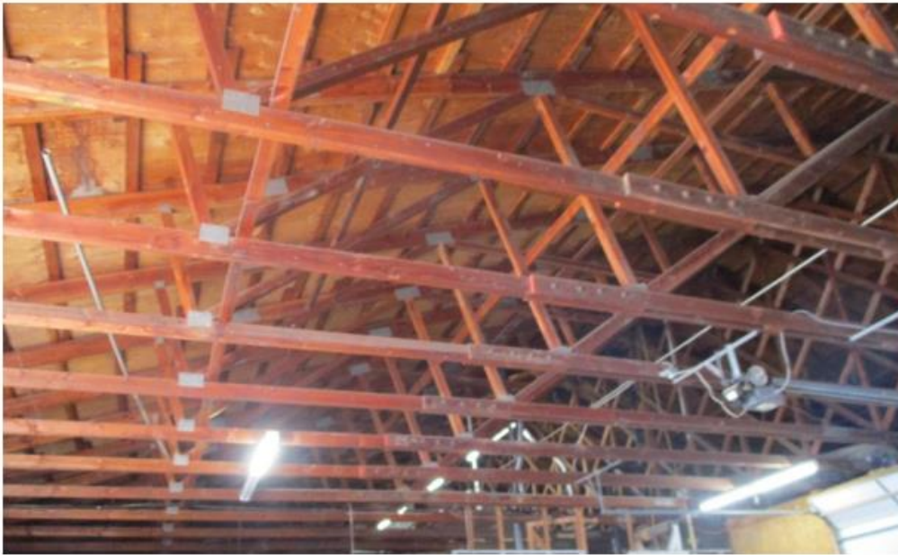
Figure 2.1. Wood Trusses Supporting Roof
