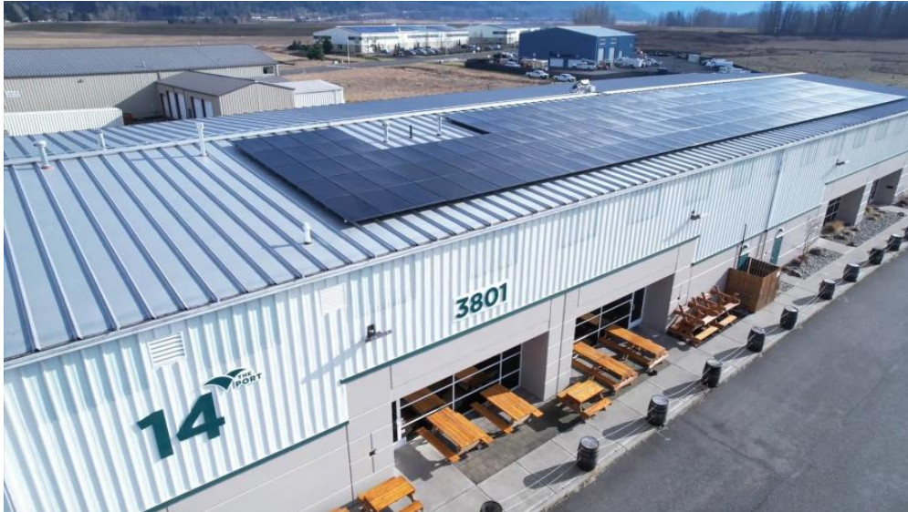
Figure 22: Clark Public Utilities installed solar panels on the roofs of five buildings, including Building 14 (above), at the Port of Camas-Washougal's Industrial Park in late 2023 and early 2024 (Flanagan, 2024).
