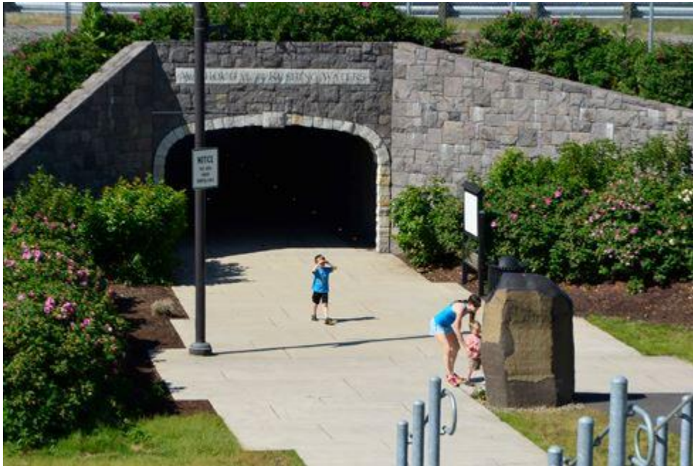
Figure 18: SR 14 pedestrian tunnel (Visit Washougal, n.d.).
