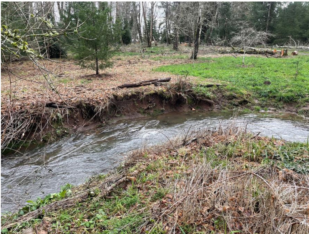
Figure 31: Campen Creek shows signs of erosion south of the pedestrian bridge in Washougal's Mable Kerr Park in 2023 (Flanagan, Washougal stormwater projects ripple out, 2024).
