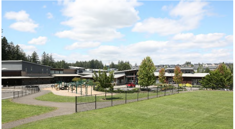
Figure 5-7 Woodburn Elementary School, Camas School District
