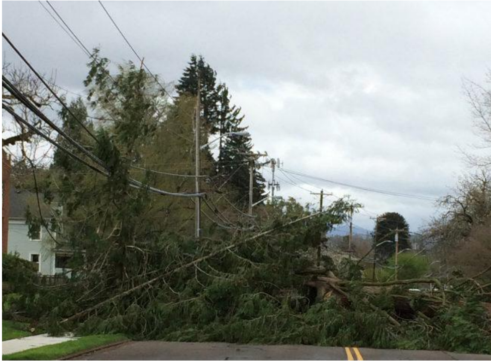
Figure 19: A cedar tree toppled during a 2017 windstorm, narrowly missing power lines on Main Street (Feldhaus, 2017).
