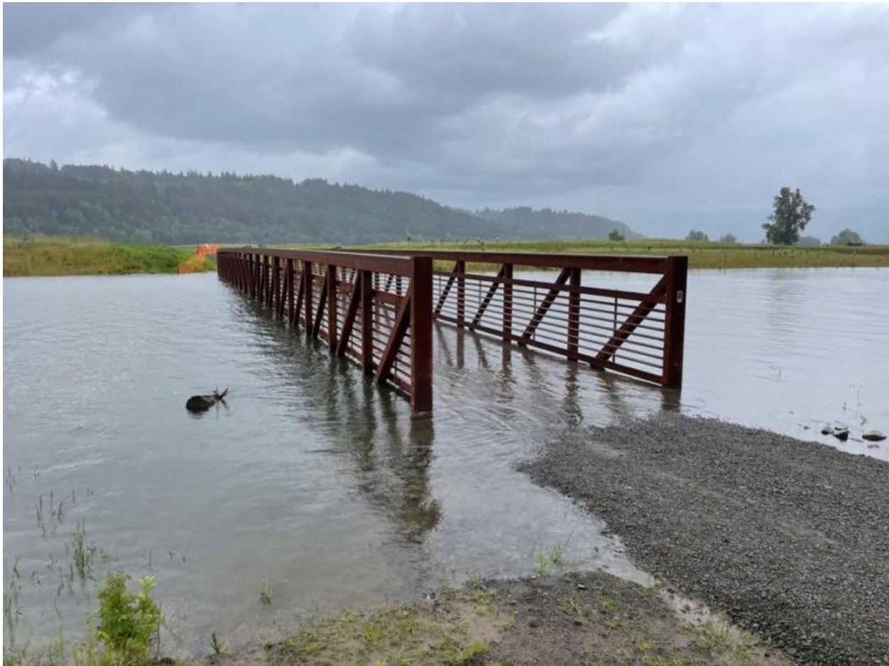
Figure 32: The newly reconnected floodplain at Steigerwald Lake National Wildlife Refuge appeared to effectively handle large rain events in June 2022, as it was intended (Flanagan, 2022).
