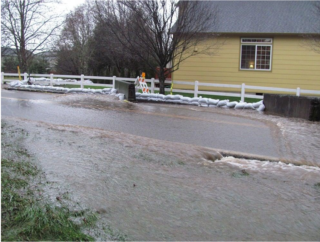
Figure 36: J Street, from 39 th to 40 th Streets, was blocked to traffic for 16 hours, due to high water on the roadway. Heavy rains and melting snow in the days prior caused culverts to overflow.
