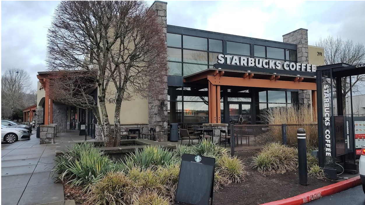
Figure 39: Rain garden and permeable pavers in the Washougal Town Center (Google Maps, 2014)
