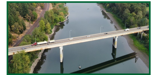
60-year-old West Camas Slough Bridge.
