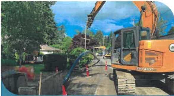
Pipe bursting limited trenching impacts while upsizing for additional capacity in this established Lake Oswego neighborhood.
