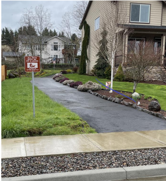
Lack of access
