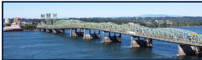
105-year old I-5 Bridge
