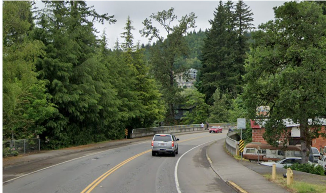
Figure 8. Facing northbound on Washougal River Road and approaching bridge crossing.
