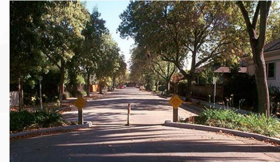
Partial Street Closure
