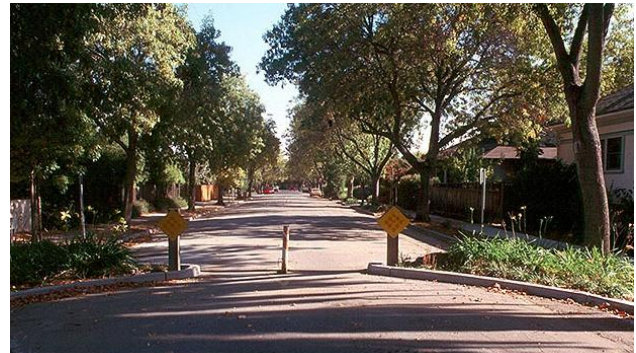
Partial Street Closure
